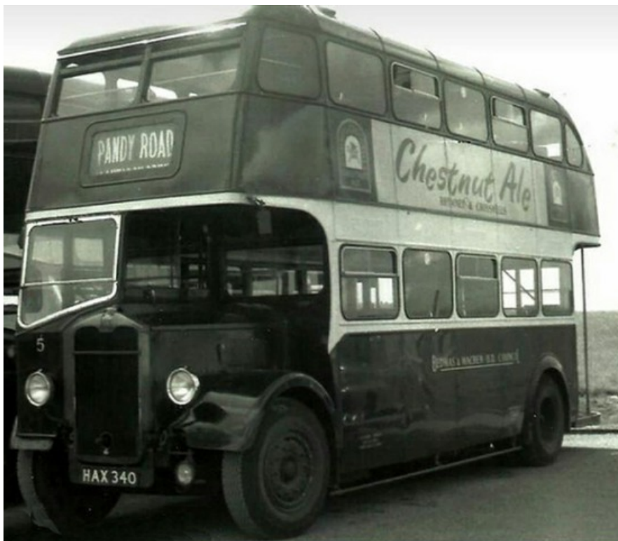
Bedwas & Machen No. 5 (HAX340) was a 1948 Albion CX1 with Welsh Metal Industries 57-seat lowbridge bodywork. It was withdrawn in 1961.
